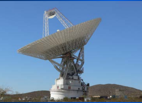
70m-Radioteleskop "Mars antenna" (1966/88-2010), Goldstone Deep Space, Kalifornien, für SETI (Search for Extraterrestrial Intelligence) (© NASA/JPL)
